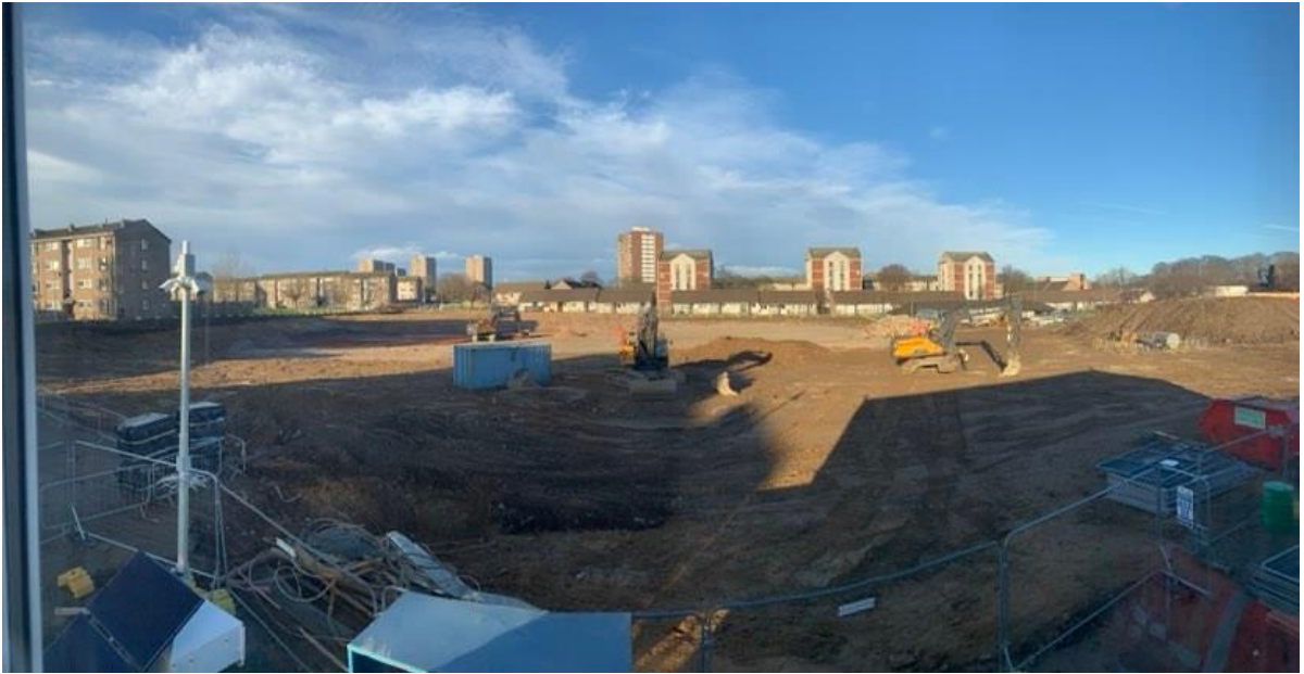
Photograph 1 – Site looking North towards Conningham Gardens and the centre of Tillydrone.
