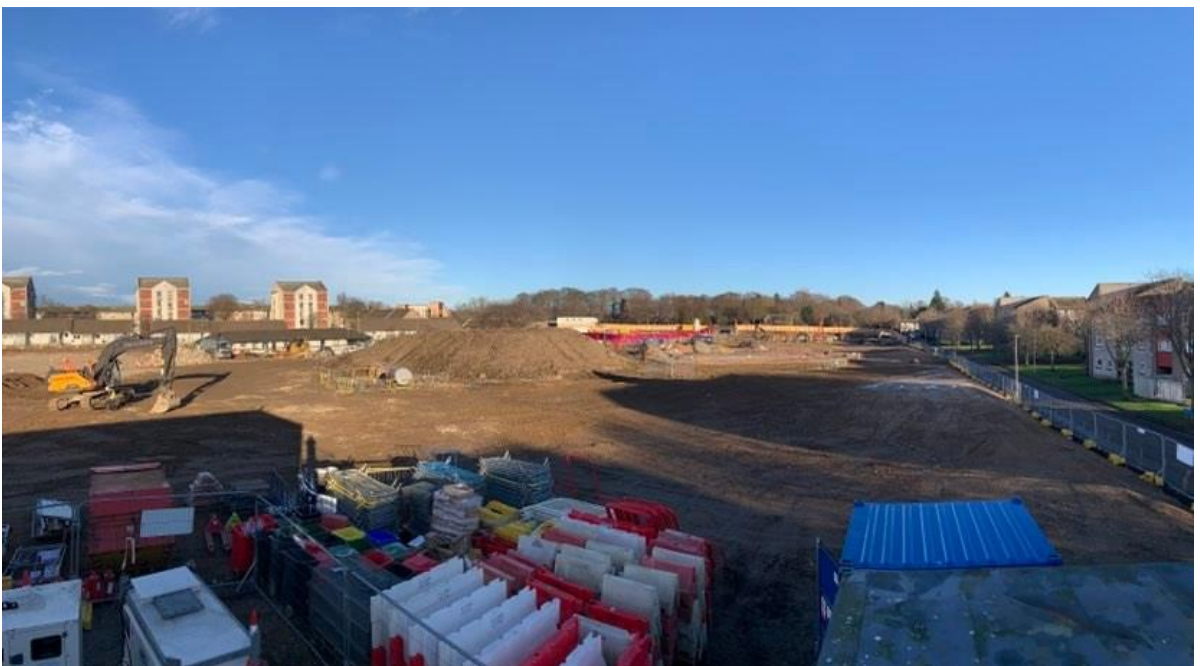
Photograph 2 – Site looking East towards Tillydrone Avenue, Harris Drive is on the right.
